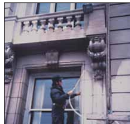
Figure 6. Spray application of silanes on large structures.
