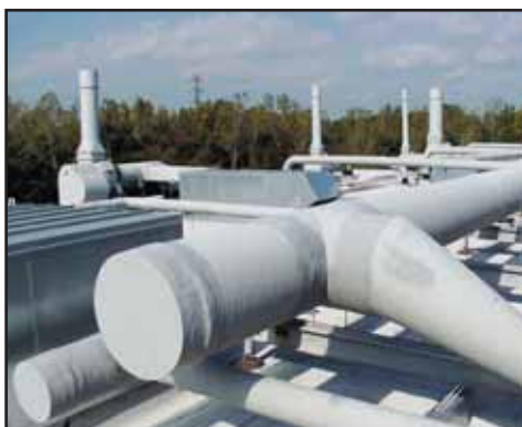
Methacrylate-silanes couple fiberglass to unsaturated polyester in corrosion resistant rooftop ductwork at Gelest, Inc.
