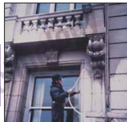
Figure 6. Spray application of silanes on large structures.
